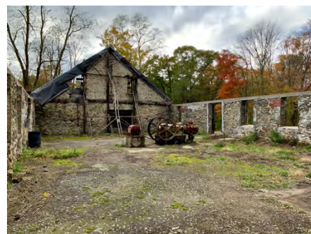
Stanley Iron Works Park, located along the Town River, was designated as a Town parkland in 1996. Listed on National Register of Historic Places since 2002, the park provides a glimpse into Bridgewater’s long history as a leading manufacturer of iron.
