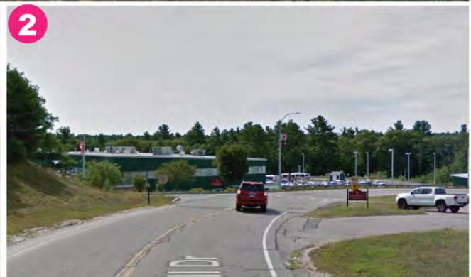
2 Lack of sidewalks and bicycle lanes on Great Hill Drive. Curves in the road also limit sight lines.
